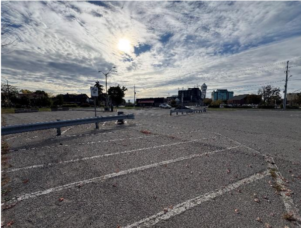
Image 3: Graded asphalt parking lot within the subject property, facing southeast
