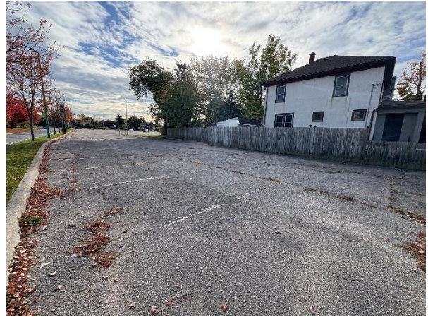
Image 4: Graded asphalt parking lot within the subject property, facing southeast
