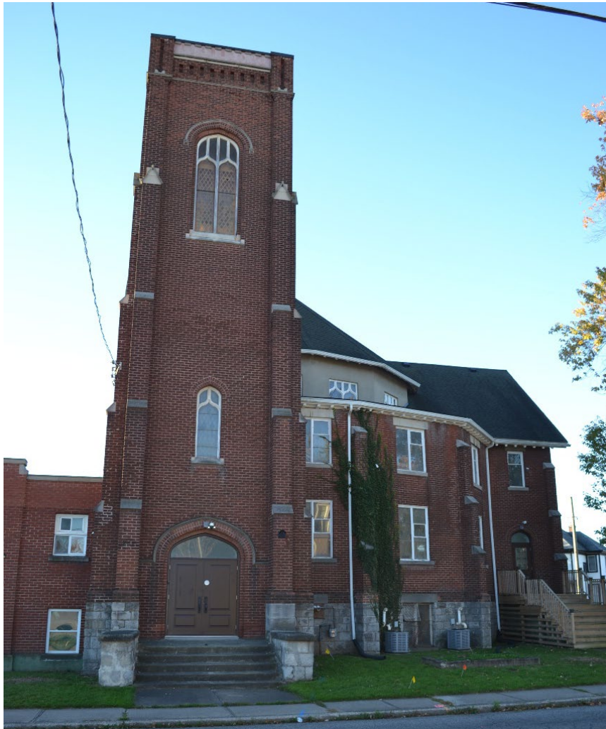
Figure 27 – The north elevation, including the main entrance (Source: PW 2025)
