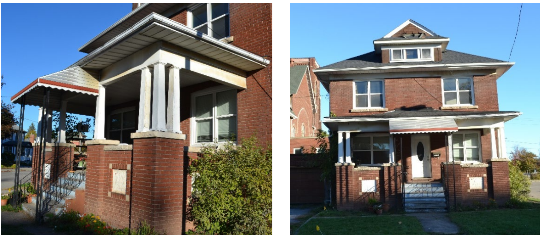
Figure 87 – The clustered columns and veranda (left) and the symmetrical façade (right) (Source: PW 2025)
