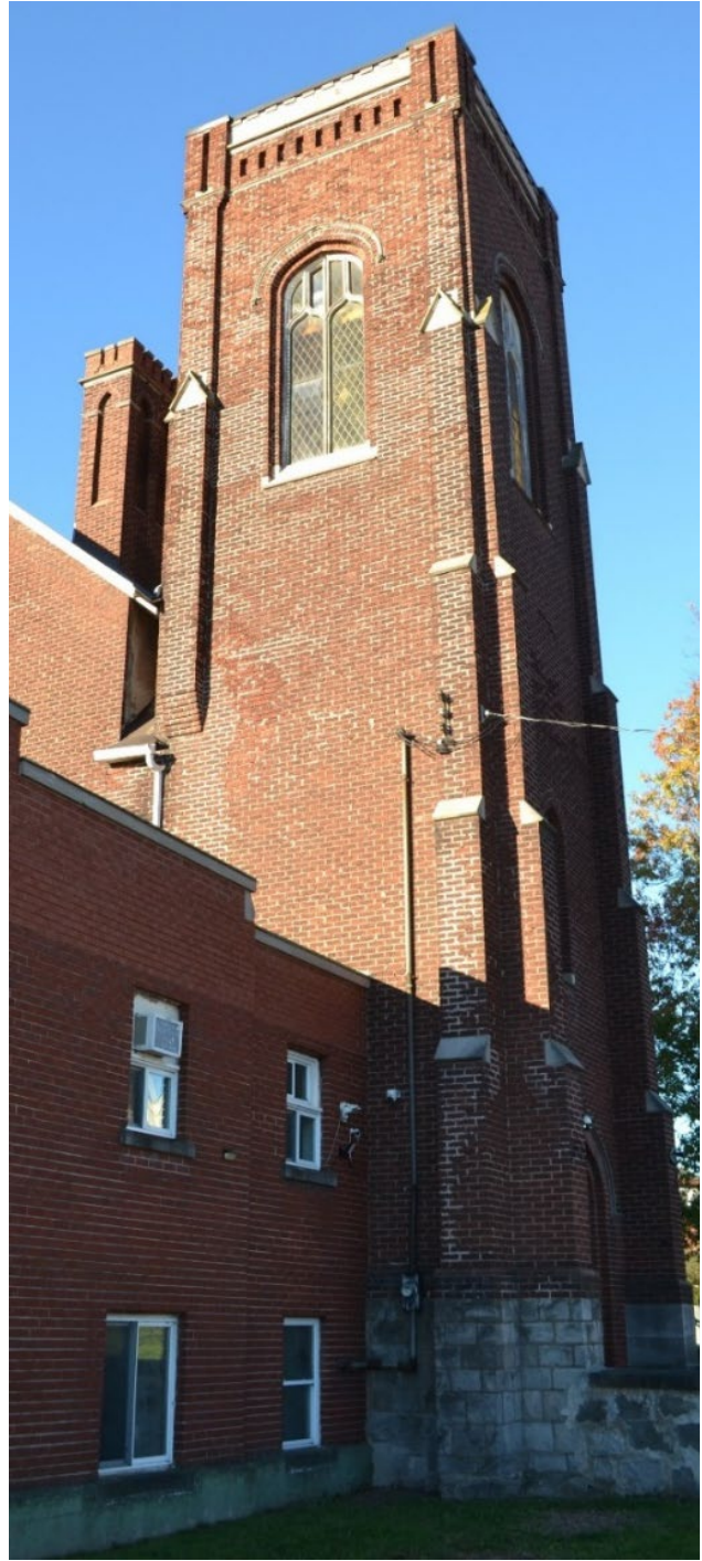
Figure 73 – Architectural features identified on the 1918 church building, such as the arched windows with tracery, window hood moulds, brick corbelling and crenelations on the chimney (top left), the rose window (bottom left), and the presence of buttresses on the tower (right) (Source: PW 2025)
