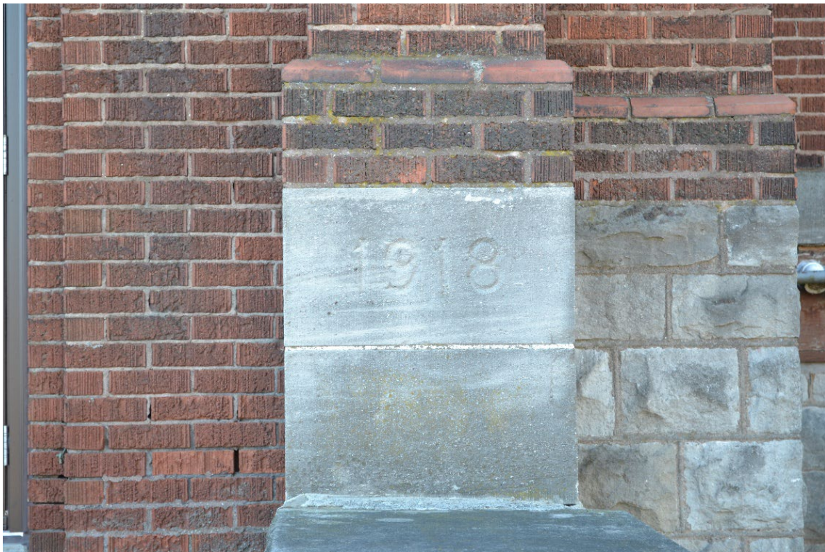
Figure 47 – The cornerstone near the main entrance to the church (Source: PW 2025)
