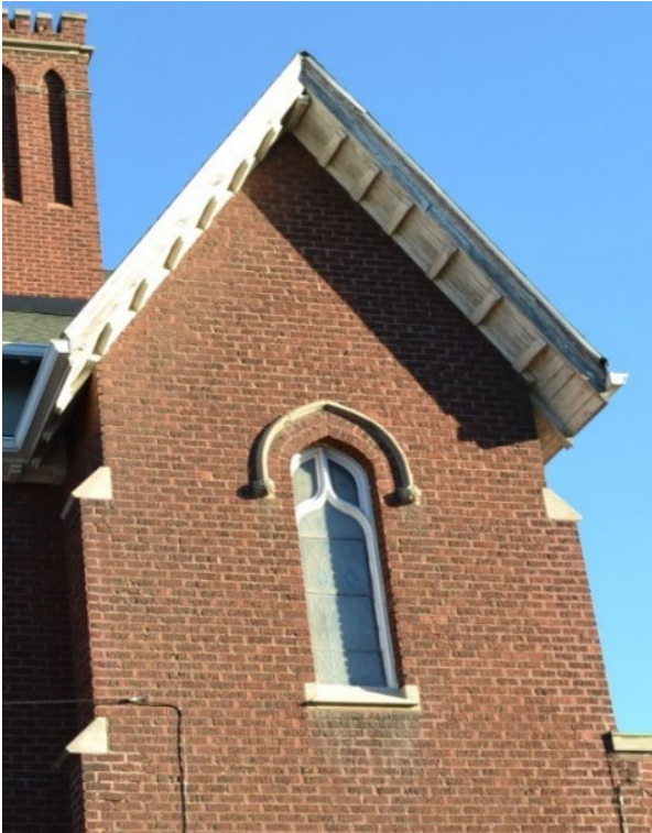
Figure 73 – Architectural features identified on the 1918 church building, such as the arched windows with tracery, window hood moulds, brick corbelling and crenelations on the chimney (top left), the rose window (bottom left), and the presence of buttresses on the tower (right) (Source: PW 2025)
