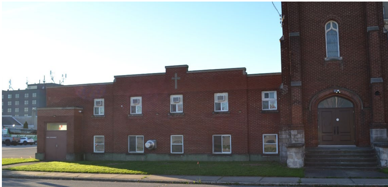
Figure 32 – The façade (north) elevation of the 1954 church addition (Source: PW 2025)
