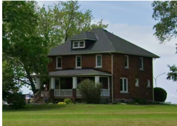
Figure 89 – Other dwellings in the neighbourhood along Kitchener Street showing Edwardian Classical forms (Source: DH 2026)
