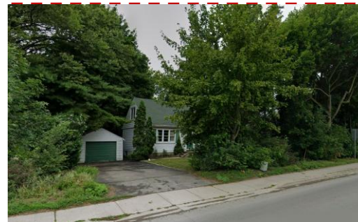
5381 MONTROSE ROAD 2-STOREYS (SINGLE DETACHED DWELLING)
