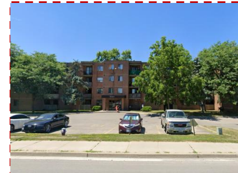
5241 MONTROSE ROAD 4-STOREYS (APARTMENT DWELLING)
