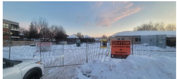
February 1, 2026 site photo
