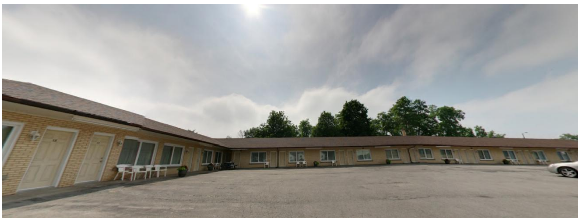
Existing motel to be renovated
