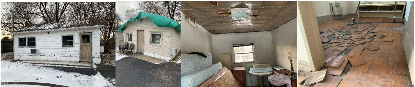
Condition of existing (now demolished) cabins on site
